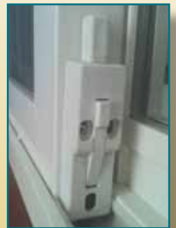
Optional dual position foot lock limits travel of sliding door.
