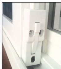
OPTIONAL DUAL POSITION FOOT LOCK LIMITS TRAVEL OF SLIDING DOOR
